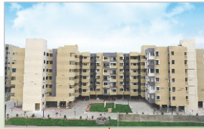
Actual Photograph of E, F Block
